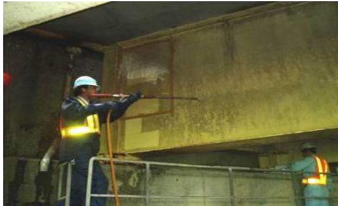
Salinity adsorbed on bridge wall before and after cleaning
