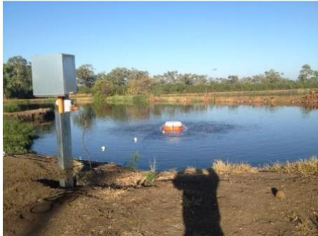
Floats are supplied with the cable as shown on the photo to the left. Cable is to be slid through the floats and spaced along the cable roughly evenly to allow the cable to easily float on the water surface.
