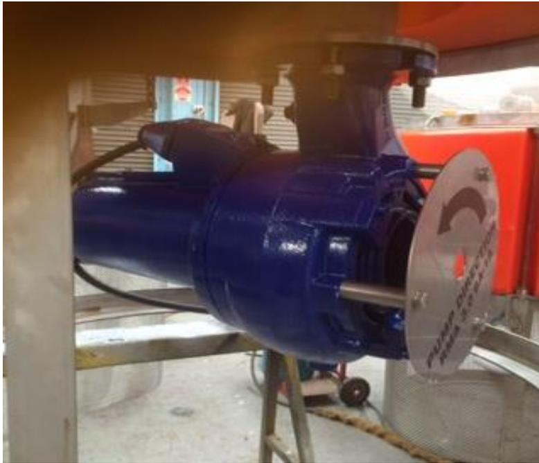
The photo to the left (RMA QA 30 model shown) shows the pump mounted below the main body of the RMA QA Unit. Note the bolts that hold the pump to the unit body. To replace the pump is as simple as unbolting four bolts, and bolting the new pump in place (remember seal). Note pump shown without screening.
